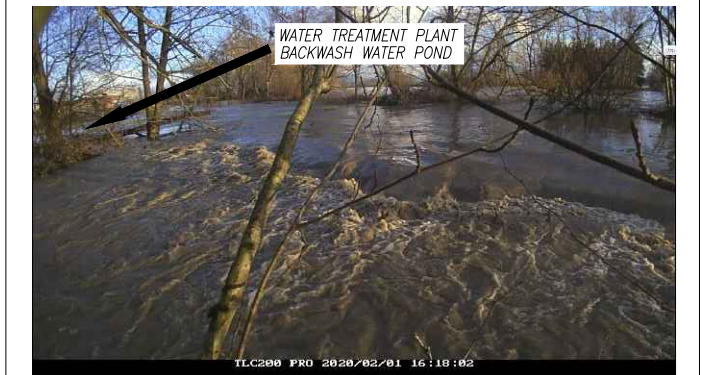
LEVEE OVERTOPPING DURING FLOOD - FEB 2020
